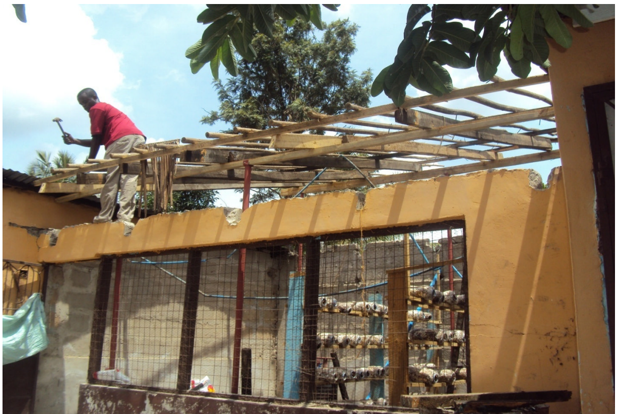
BELOW: After pulling down the old roof, the building's height is raised to acceptable standard.
