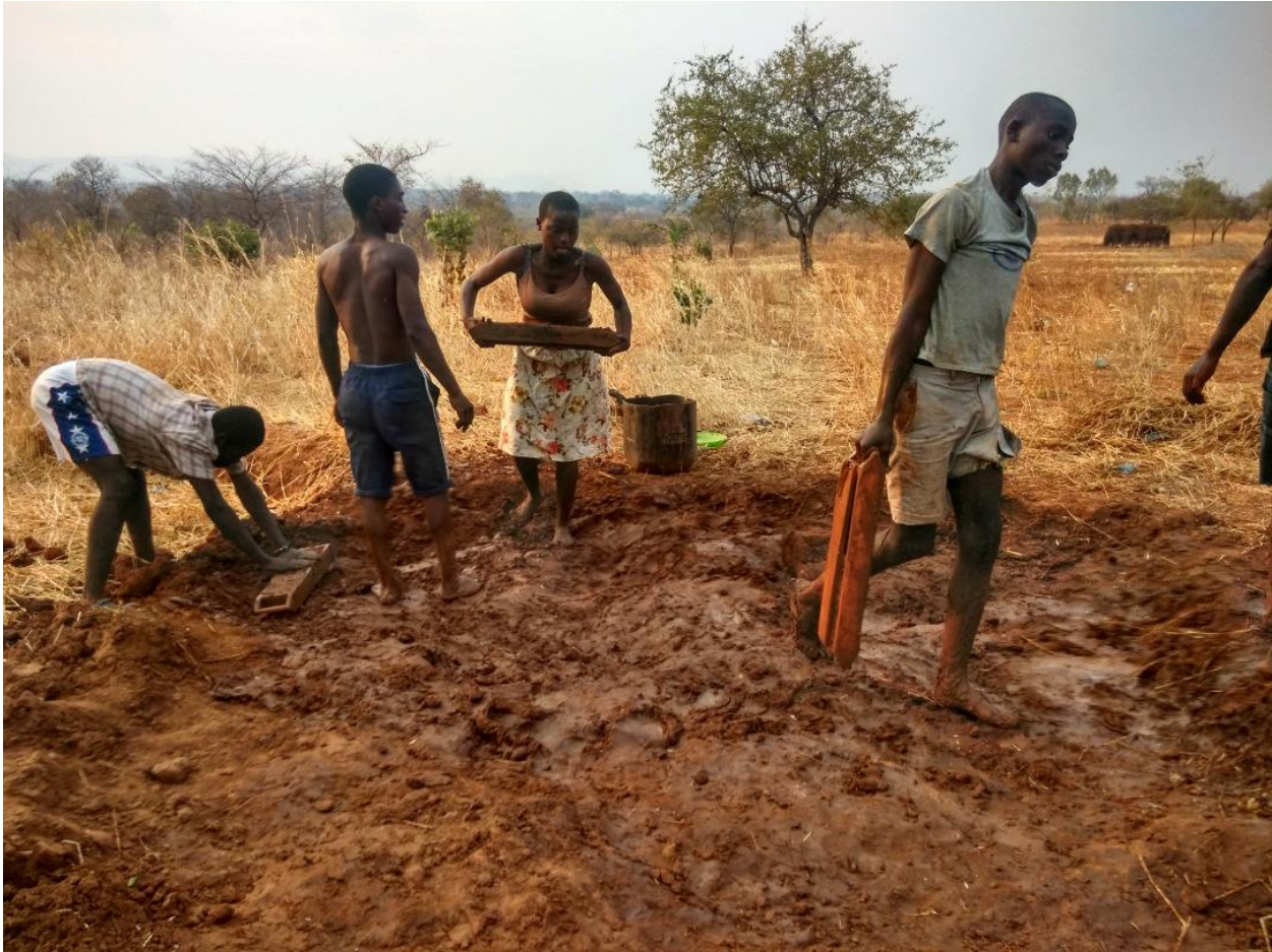
The community also moulded bricks for construction
