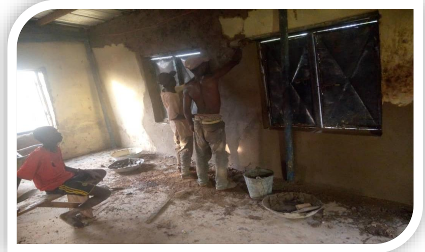
Plastering of walls and floor. And extended the workplace to make way for a water
