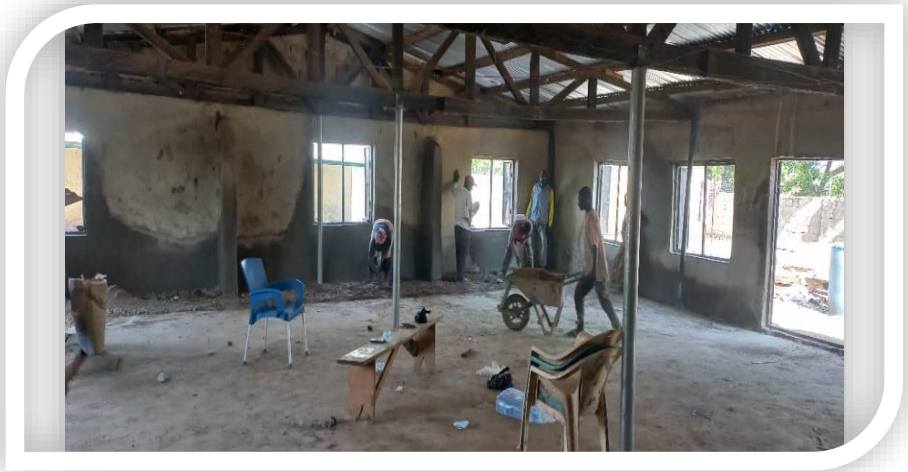
75 mm diameter metal poles/ pillars inserted to support roof.
