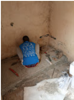
Before floor tiling_compress50.jpg 347K
