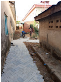
Interlocks in toilet area_compress20.jpg 524K
