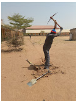
Connecting pipes to water source_compress30.jpg 565K
