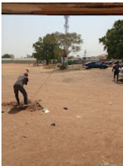
Connecting pipes to water source 1_compress21.jpg 569K
